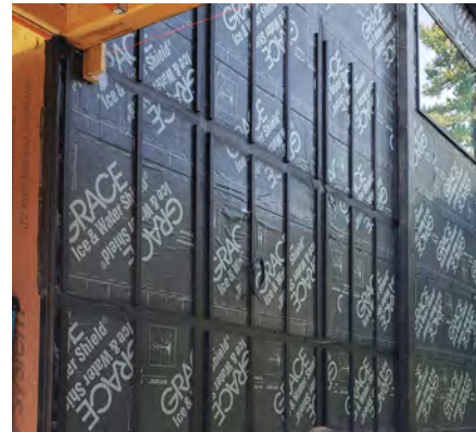
Cor-A-Vent Furring Strips installed and ready for panels.
