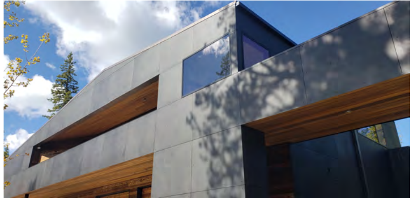
Sandblasted Black Stainless Steel panels with oil & wax will not rust and maintains the original finish longer.
