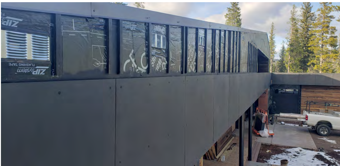
Furring Strips placed to line up with screw holes of metal panels for mounting.
