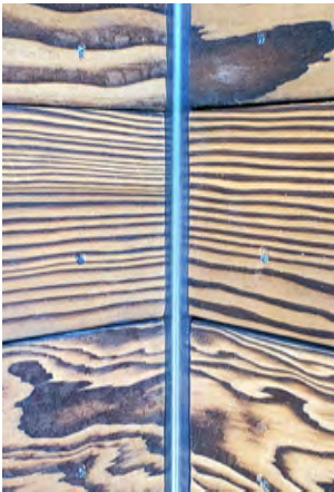
Figure 3.1 WD/WD Inside Corner
