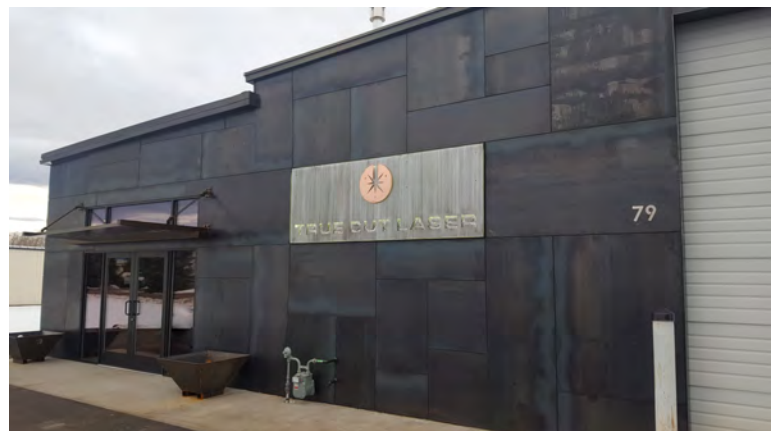
The front of True Cut Laser shown with Blackened Hot Rolled panels laser cut to various shapes and sizes. 1/4" reveal between all panels.
