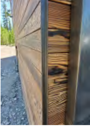
Figure 1.1 WD/WD Outside Corner
