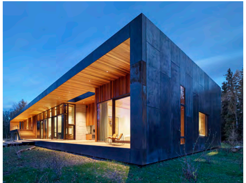
Blackened Hot Rolled Steel panels with oil & wax showing weathered appearance after a number of years. Cold & Hot Rolled Steel would require a sealer to resist rusting.
