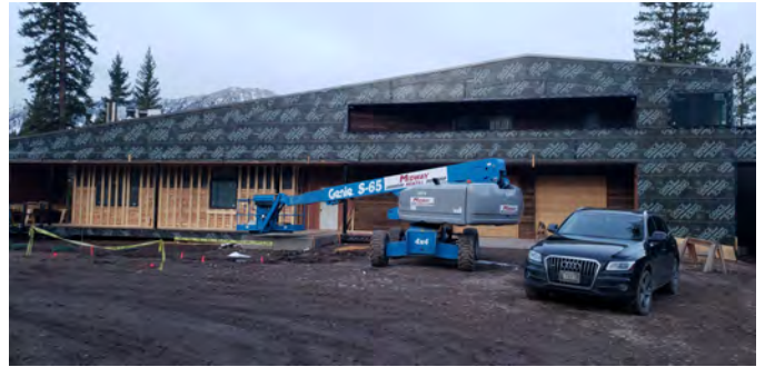
Grace Waterproof membrane shown before furring strips and panels installed.
